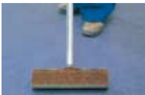
Rubbing down the sheets with a rubbing iron, a device covered with needle felt...
