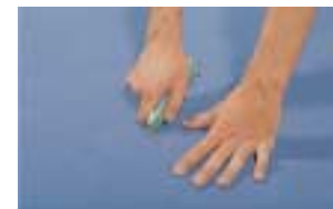
A useful tip if the trapped air cannot be forced out laterally: make a small hole with the point of a blade in a dark section of the pattern, press out the air and once again firmly rub down the covering at this point.
