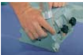
Milling out the joint.
