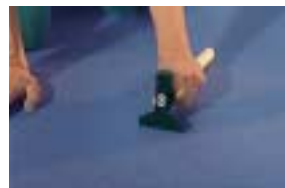
Remaining air bubbles should be rubbed down with an appropriate smoothing tool.
