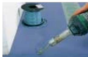
Sealing with a manual welder.
