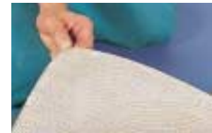
Adhesive must be applied in such a way that the strips of adhesive cover the entire backing of the floorcovering.
