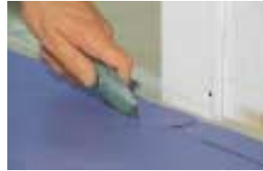
The floorcovering is cut along the scored contours.
