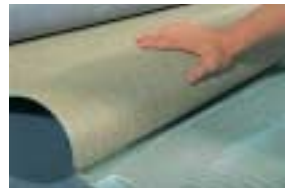
Folding back the trimmed sheets, either half-way back in the case of rooms or lengthways in the case of corridors etc...
