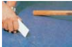
The seam should never fit too tightly. There should be a space of approx. 0.5 mm between adjoining edges when sealing.
