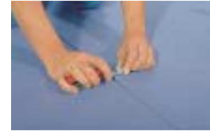
The safest way of cutting a seam: mark the top sheet with an under and over scriber guided along the trimmed edge.
