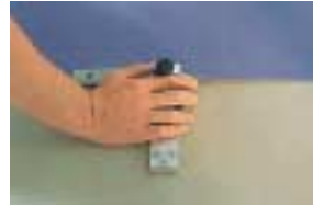
Cutting the first edge of the sheet is best done with a linoleum edge cutter or strip trimmer.
