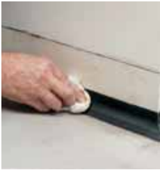
Coat the floor with acrylic adhesive to within 10cm of the wall then lay the Chocflex sheet.
