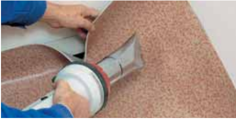
To facilitate adhesion in the curves, warm the floorcovering. Cut into the corners of the walls, beginning at the base of the wall at an angle of 45°.
