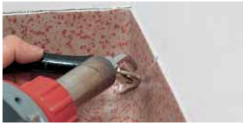
Hot weld the seams.
