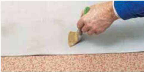
Fold back the edges of the sheet and apply contact adhesive to the back of the material and to the wall up to the pencil mark. Press the sheet firmly into place.
