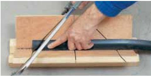
Ensure that covings are clean and free from grease and cut them to the required lengths.
