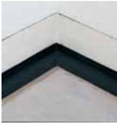
Coat the floor with acrylic adhesive to within 10cm of the wall then lay the Chocflex sheet.
